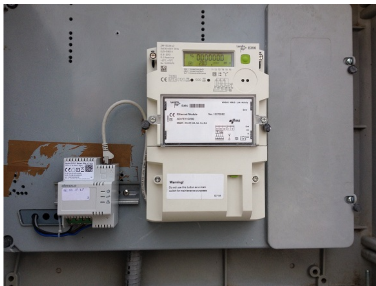
Figure 2 - Meter cabinet with the G3-PLC DINRail modem (on the left) connected to the smart meter (on the right)
